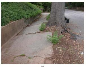
Figure 30.31 With heights nearing 116 meters, (a) coastal redwoods (*Sequoia sempervirens*) are the tallest trees in the world. Plant roots can easily generate enough force to (b) buckle and break concrete sidewalks, much to the dismay of homeowners and city maintenance departments. (credit a: modification of work by Bernt Rostad; credit b: modification of work by Pedestrians Educating Drivers on Safety, Inc.)
